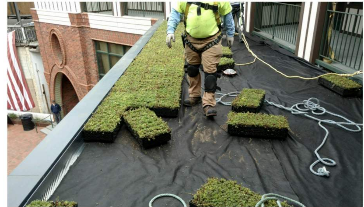
MODULAR PLANT TRAYS GREEN ROOF REFERENCE
